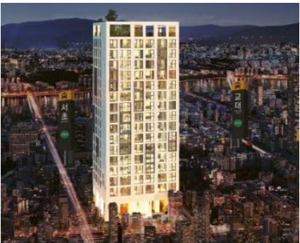
Seocho Office Building (DSME Construction)
