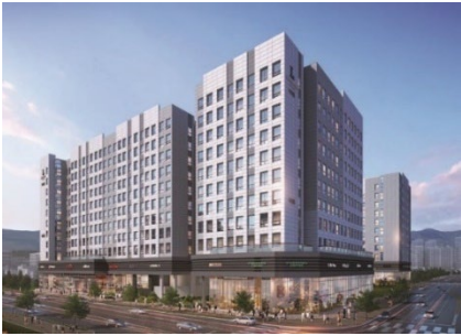
Okjeong Office Building (Daehan Construction)
